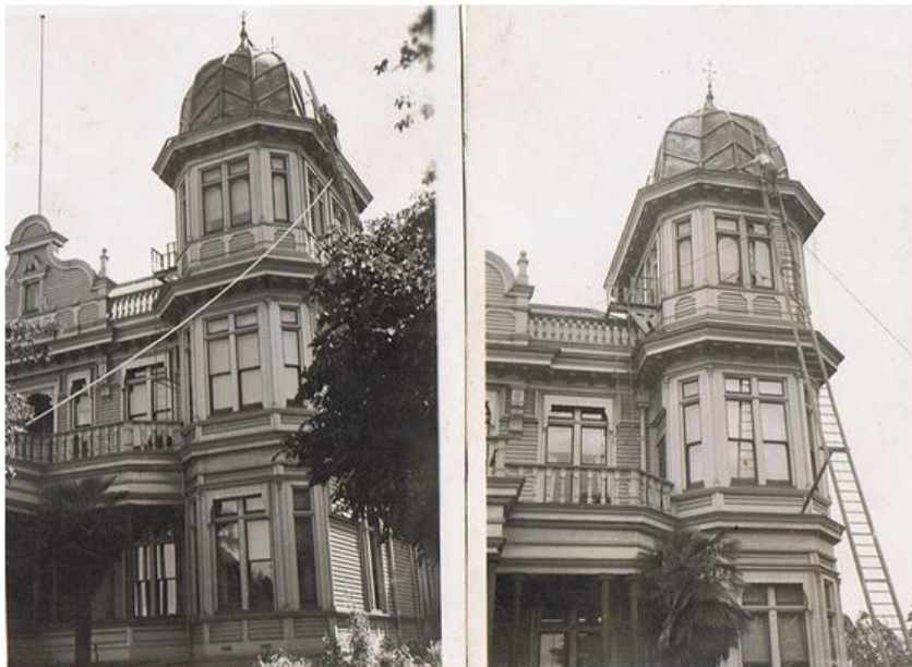
George_LeBrun_up_ladder_at_McLean_institute_building_Manchester_St_ChCh , CC BY-NC-SA 3.0 NZ. Kete Christchurch. Entry in the 2014 Christchurch City Libraries Photo Hunt by Sandra Serra.
