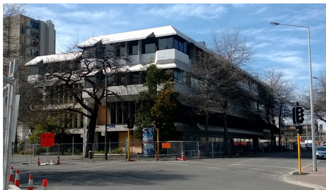
The Warren and Mahoney designed Central Library on the corner of Oxford Terrace and Gloucester Street opened in 1982. By 2008 this was too small. And it was damaged in the 2011 earthquakes.
