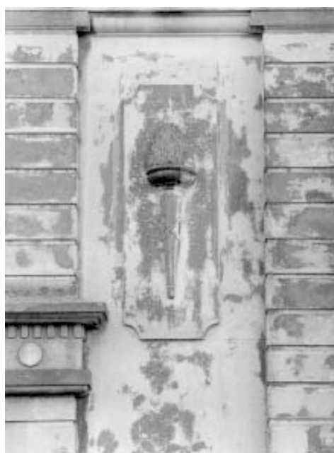
Milton Street Substation, detail of torchere
