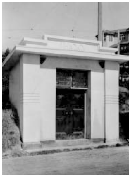
Dyers Pass Road Substation, 1929
