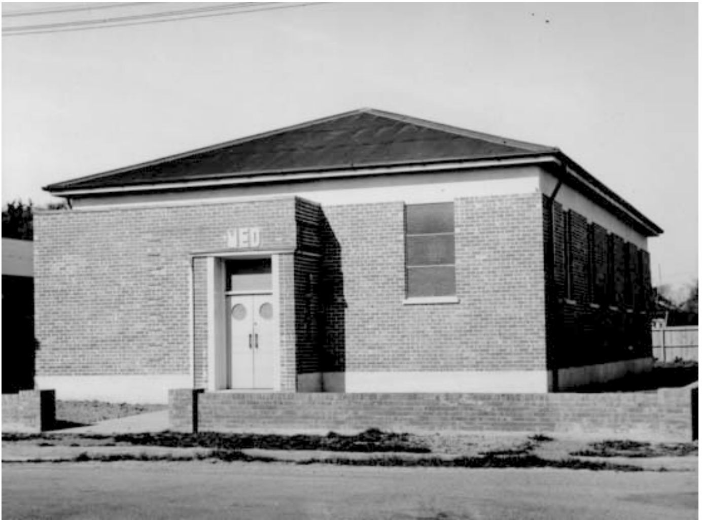
Corner Weka and Tui Street Substation
