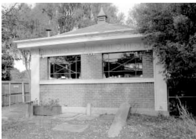
Matai Street, Pump No. 24
