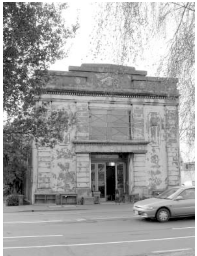
Milton Street Substaion
