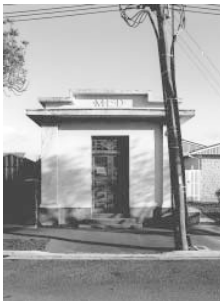
Gamblins Road Substation
