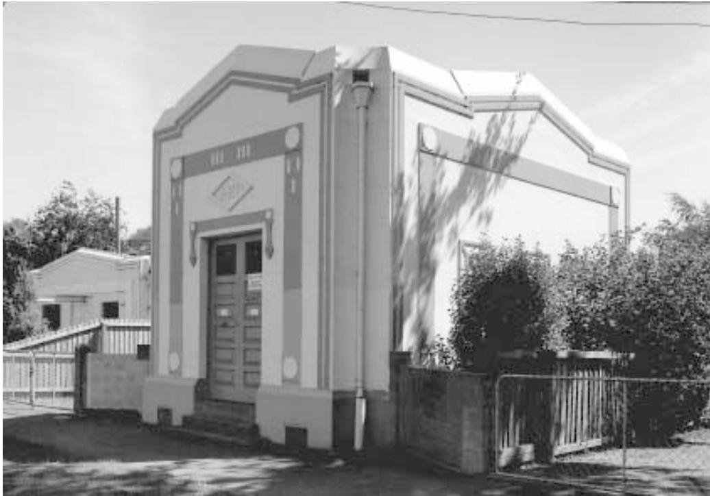
Retreat Road Substation
