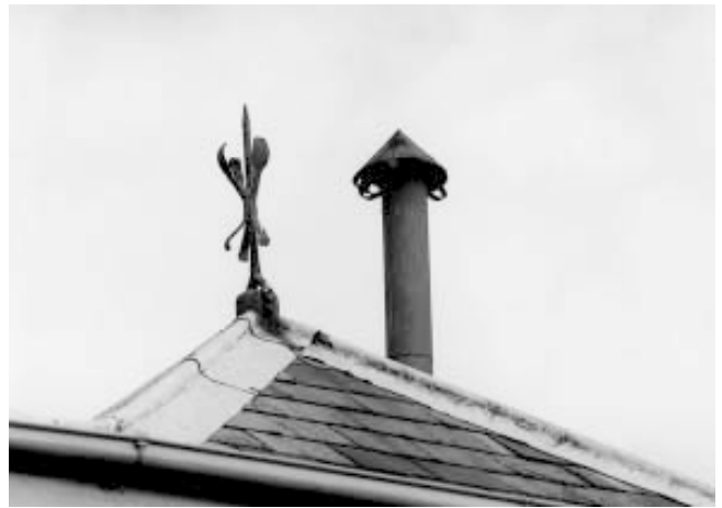
Templar Street No.4 Pump detail
