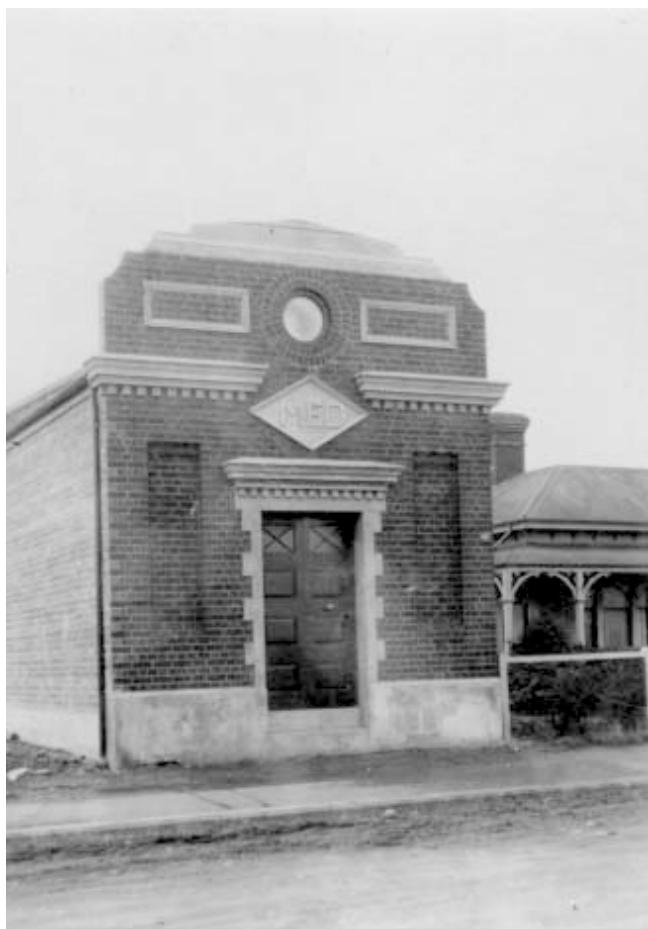
Canal Reserve Substation
