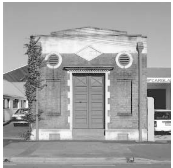
Gasson Street Substation
