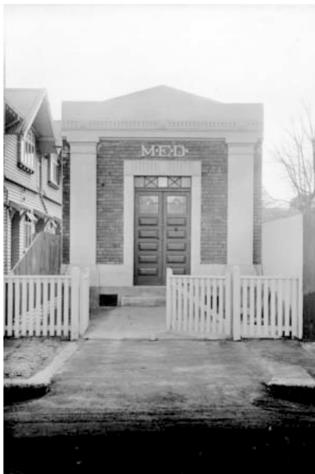
Worcester Street Substation
