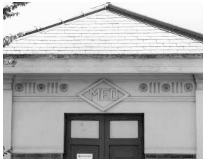
Detail, Woodham Road Substation
