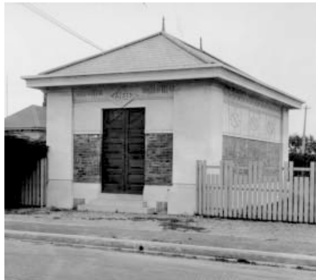
Woodham Road Substation
