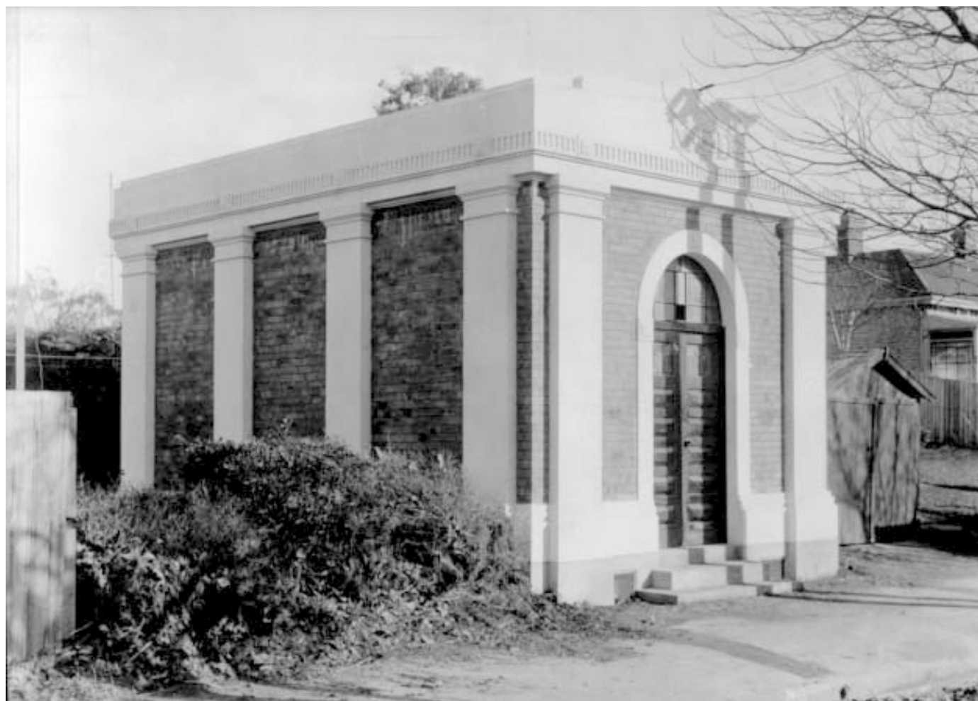
Linwood Avenue Substation just after completion in May 1935
