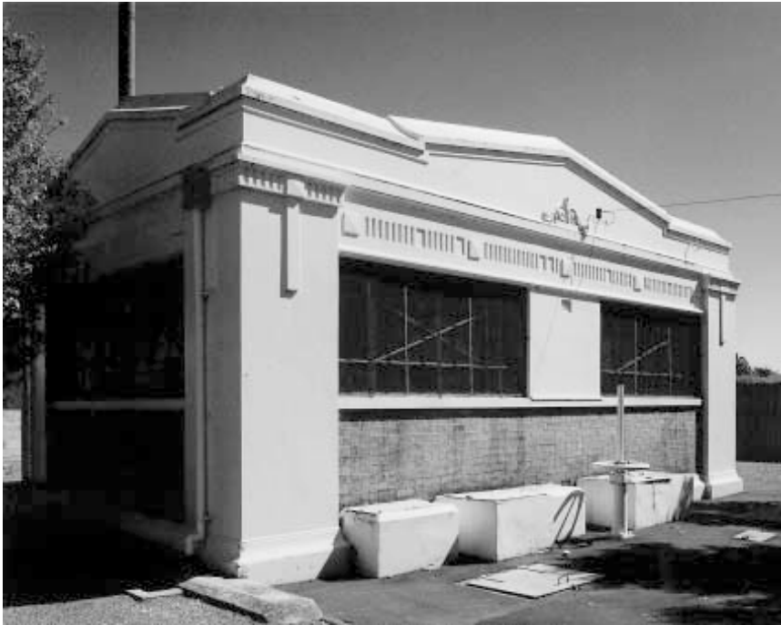
Randolph Street, Pump No.11
