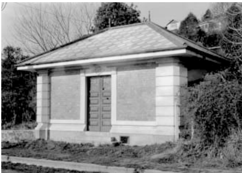
Vernon Terrace Substation, August 1944
