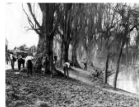
R B Owen's navvies working on the banks of the Avon, 1920s. Hocken Library
