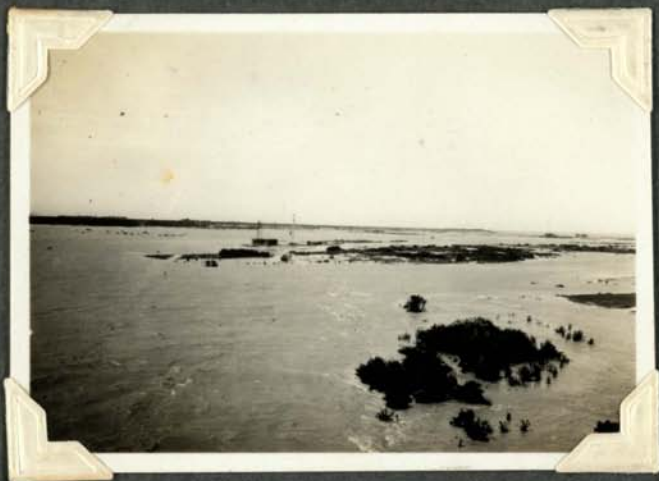
View from bridge looking downstream. H pole & cylinders isolated in centre of river. Main stream on left.
