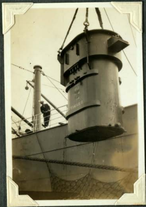
1 st Transformer on slings being lowered to truck.
