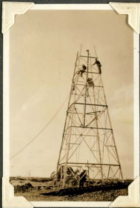
Tower N o 158. 55 Ft. suspension under construction.
