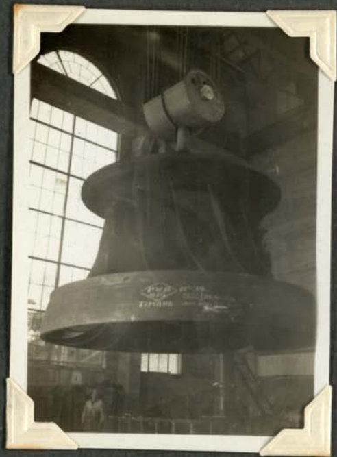
N o 2 Turbine runner on crane.
