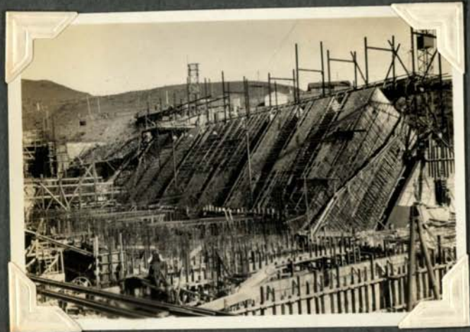
Showing penstocks and reinforcing.
