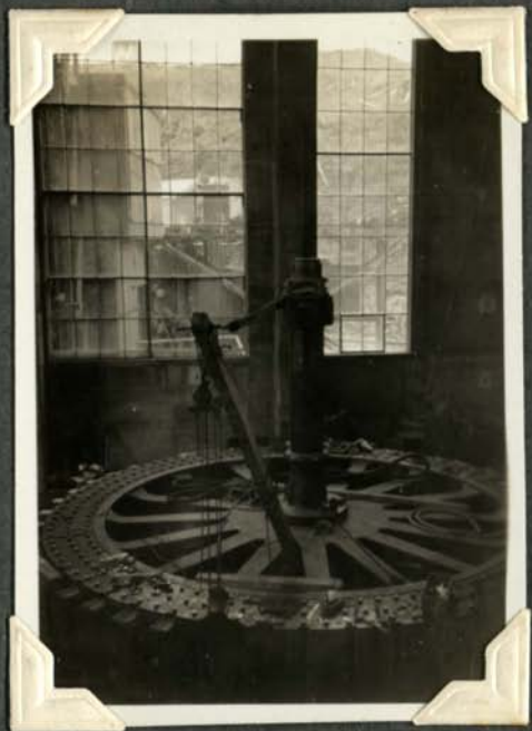
Rotor for N o 2 generator. Core plates assembled & field poles being fitted.
