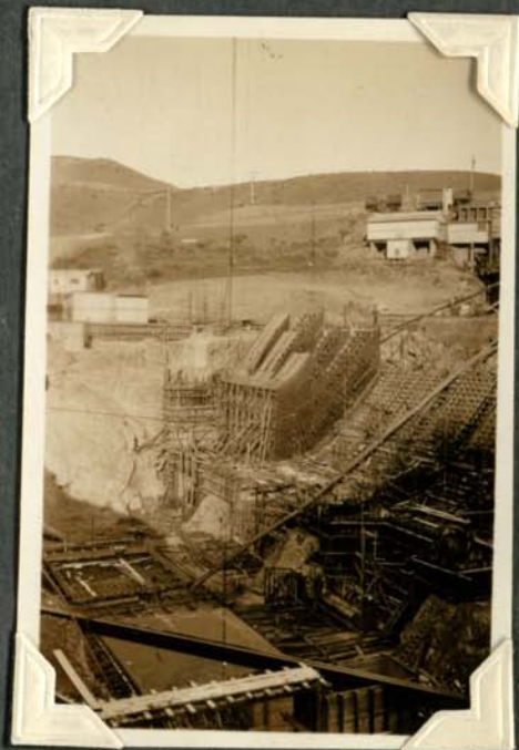
Powerhouse formwork. Penstock forms for No 5 unit being placed.
