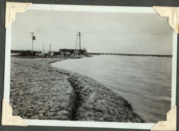
First row of netting around temporary structure dropping and protecting bank by forming an apron.
