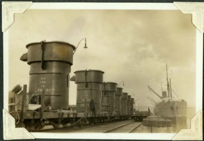
All 7 transformers on trucks, S.S. Port Pirie at wharf.
