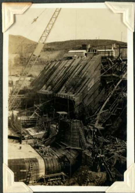
Powerhouse. No 2 Draft tube in position.
