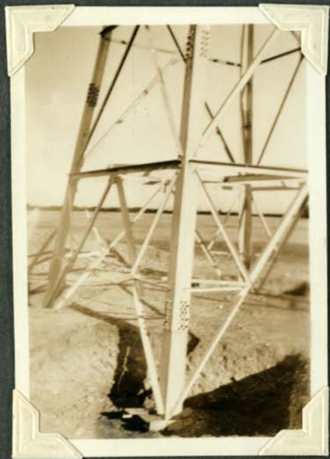
Waitaki-Glenavy Line. Footing of terminal tower at Substation site.
