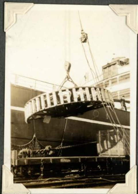
N o 2. Generator half rotor spider.
