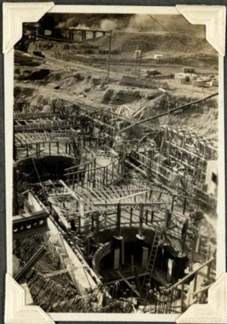
Looking down on Nos 1 + 2 turbine pits. Guide vanes in position.
