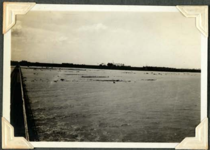
View looking towards Glenavy. Steel towers on far bank faintly visible
