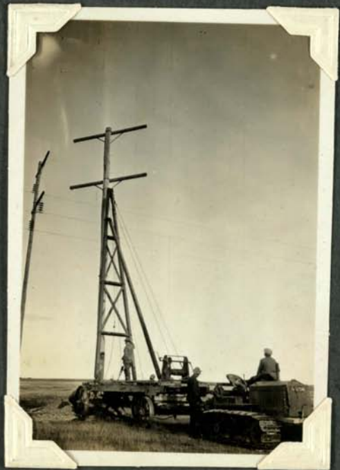
Cletrac tractor and portable crane lifting 52 Ft. pole
