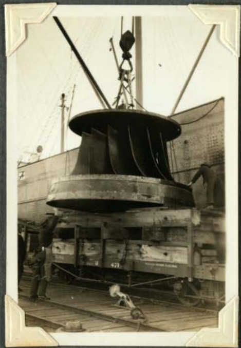
Runner being centred on truck.
