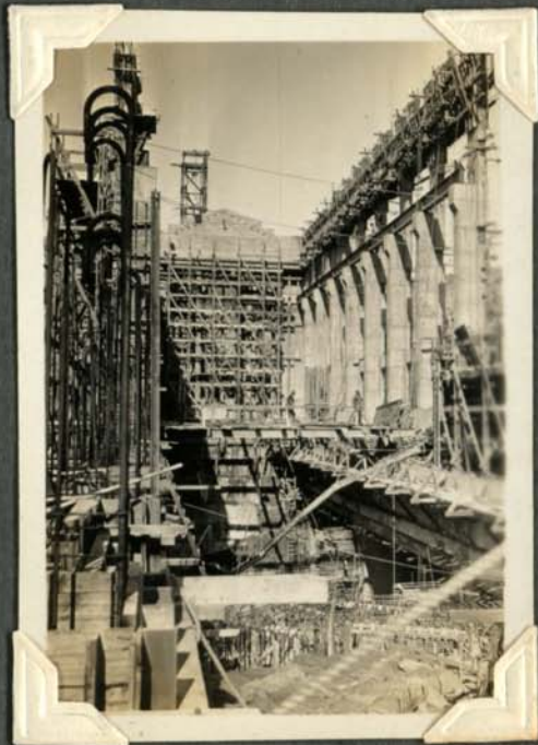
Crane runway in position on West wall of generator room.
