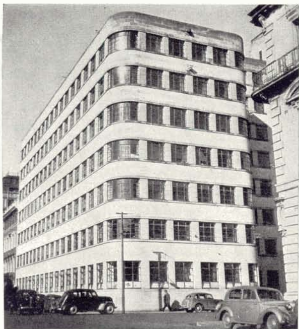
Government Departmental Building, Wellington, designed by Public Works Department. The structural steel frame is faced with local stone
