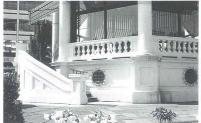
Stairs, balustrade and circular window
