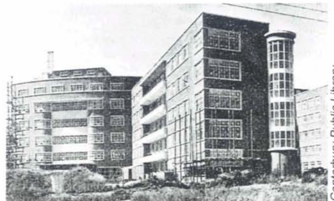
The Princess Margaret Hospital under construction
